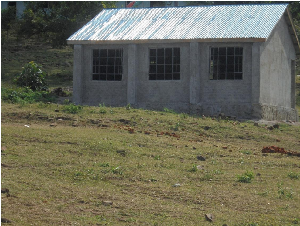
The renovated classrooms at both Kugitura and Sorore Primary schools.
