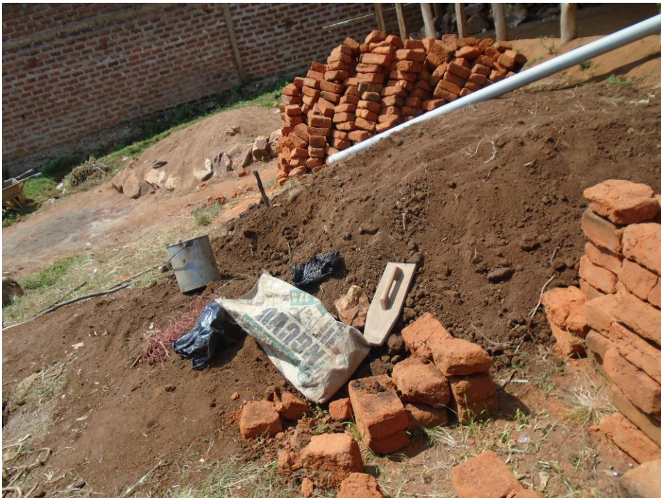
Progress of the VIP latrines
