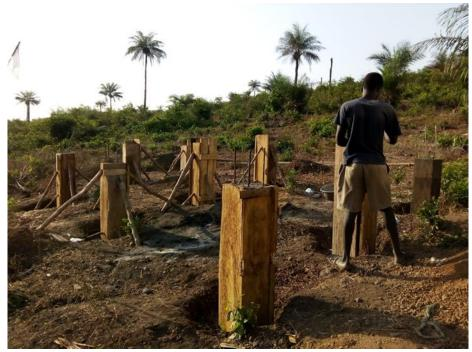
Work progressed in constructing the pen on concrete pillars, leaving ample space under the structure to allow the group to collect goat droppings to be used as fertilizer for the vegetable plots.
