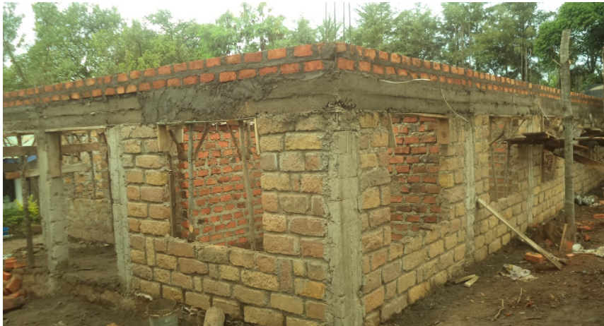
Walling at its last stage (wall plate) to roofing
