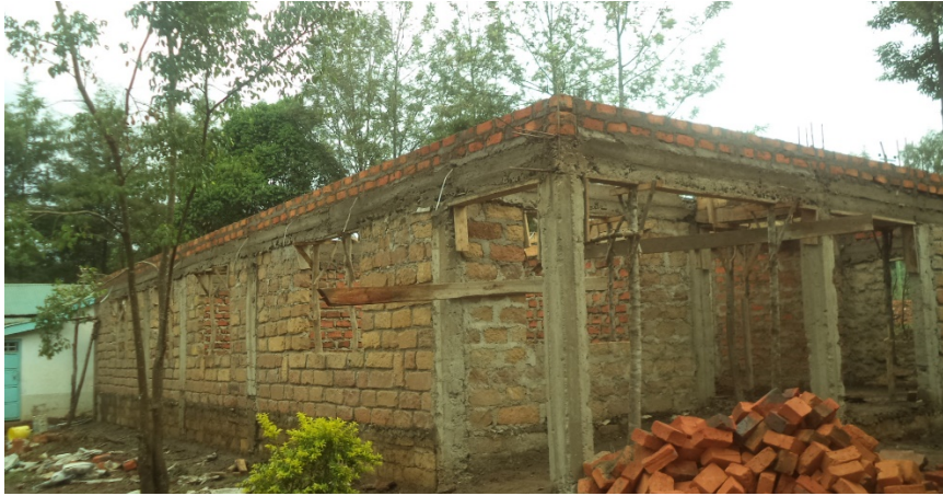
Walling at its last stage (wall plate) to roofing
