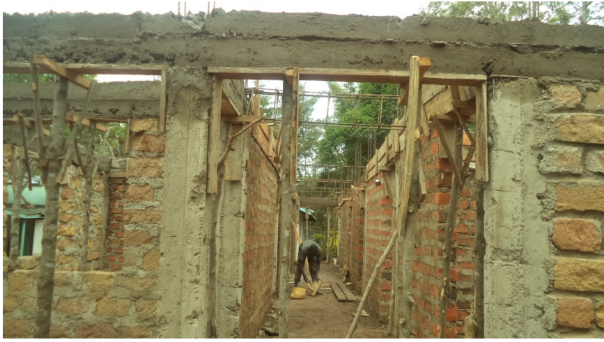
Walling-Ring beam level
