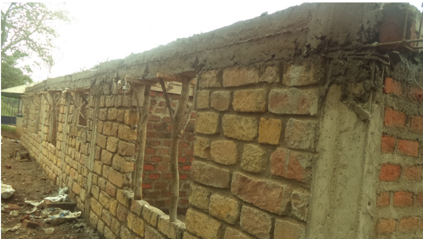
Walling-ring beam level
