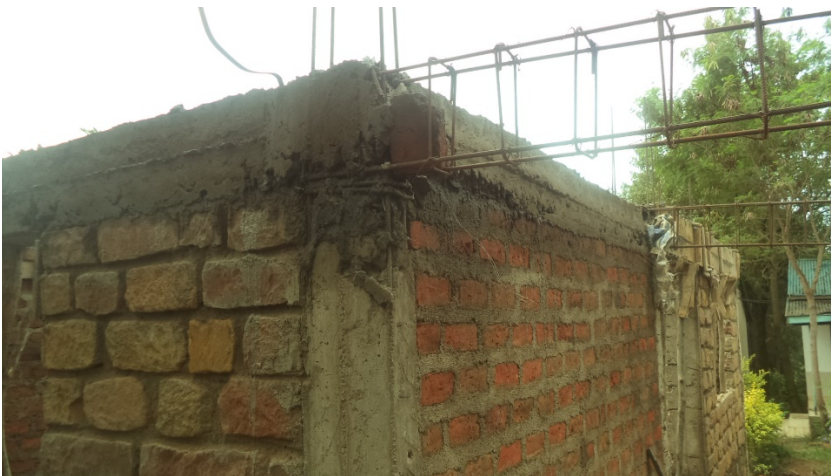
Walling- Ring beam level
