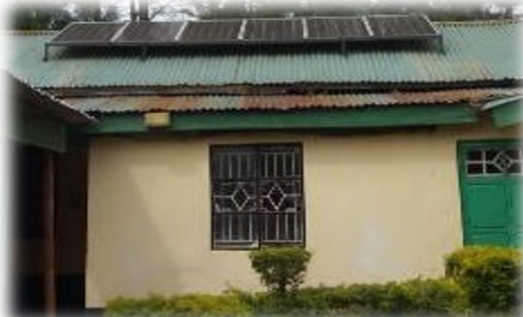
Figure 4: Installed Solar Power System (Solar panels and Invertor) to run the pump
