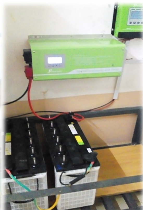
Figure 4: Installed Solar Power System (Solar panels and Invertor) to run the pump
