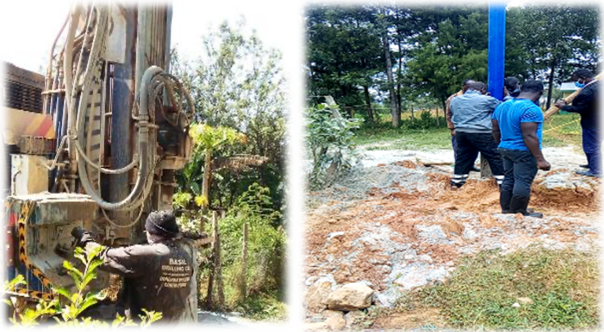
Figure 1: Drilling and Casing Process.
