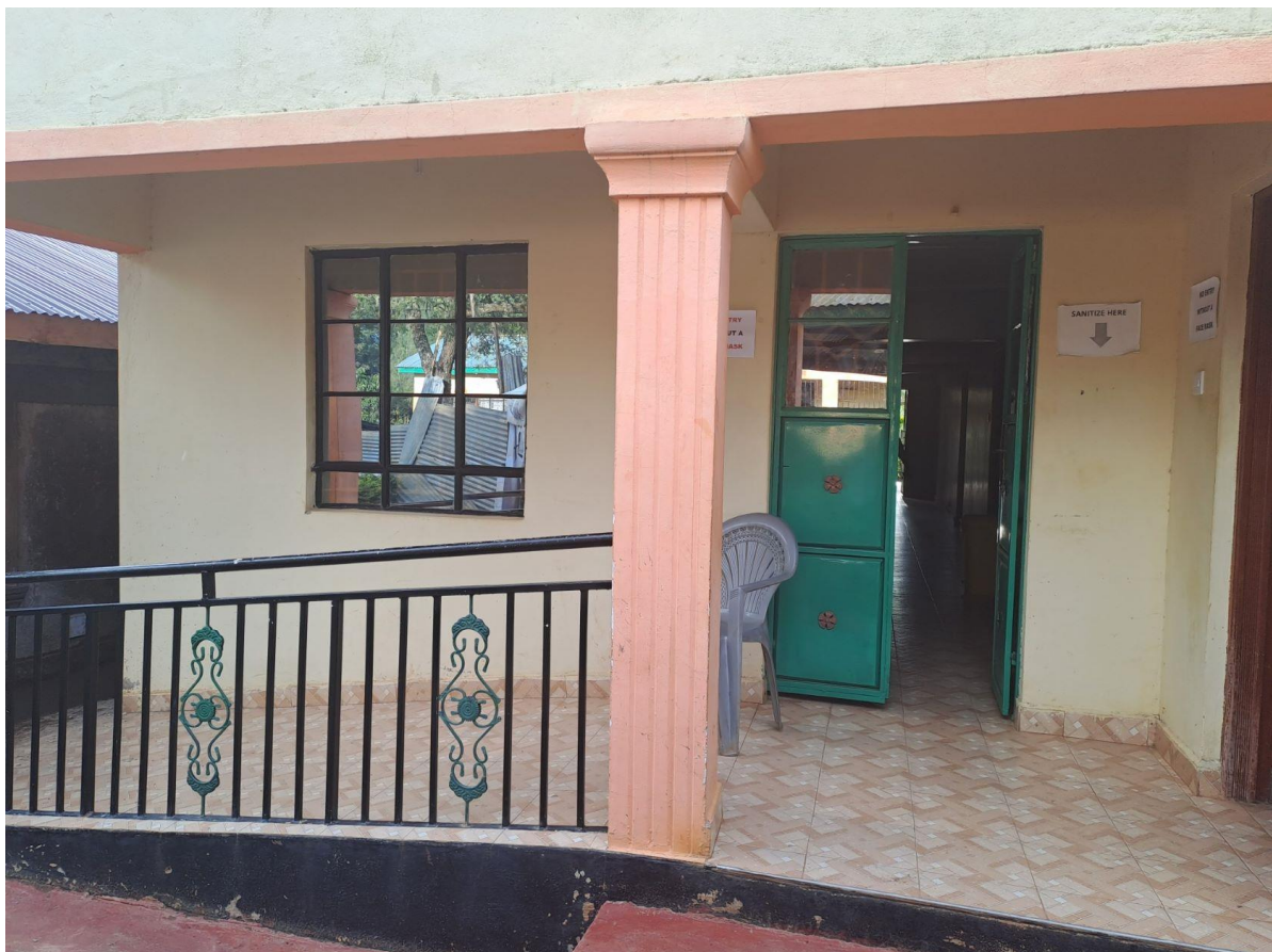
The main entrance of the Modern Maternity.
