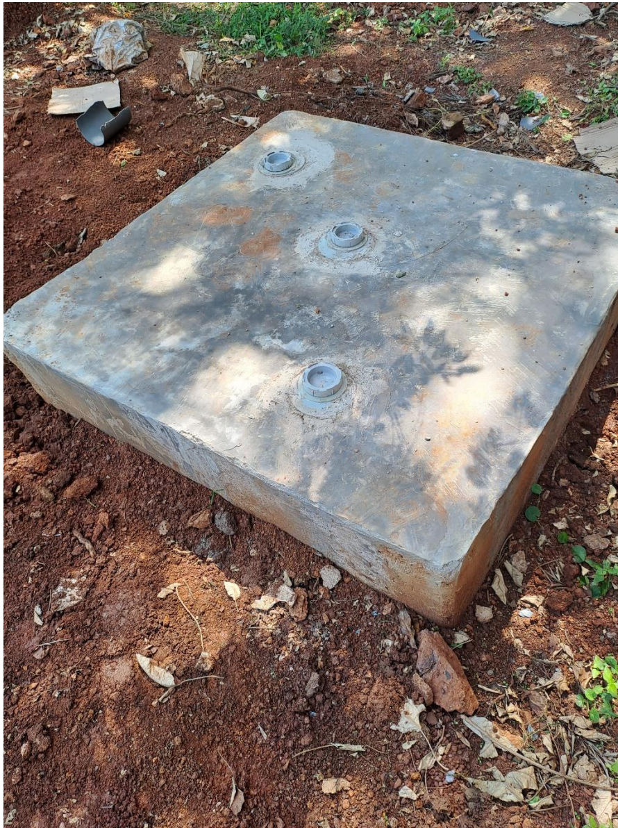
Final stage of the biodigester closed.
